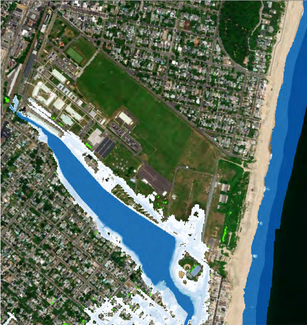
Figure 3. Sea Girt National Guard Training Center with a Total Water Level of 3 ft.
